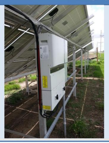
Wire in / out of inverter may be required to be in conduit.
