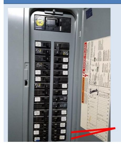
Panel is usually maxed out Need to make room Double up smaller breakers
