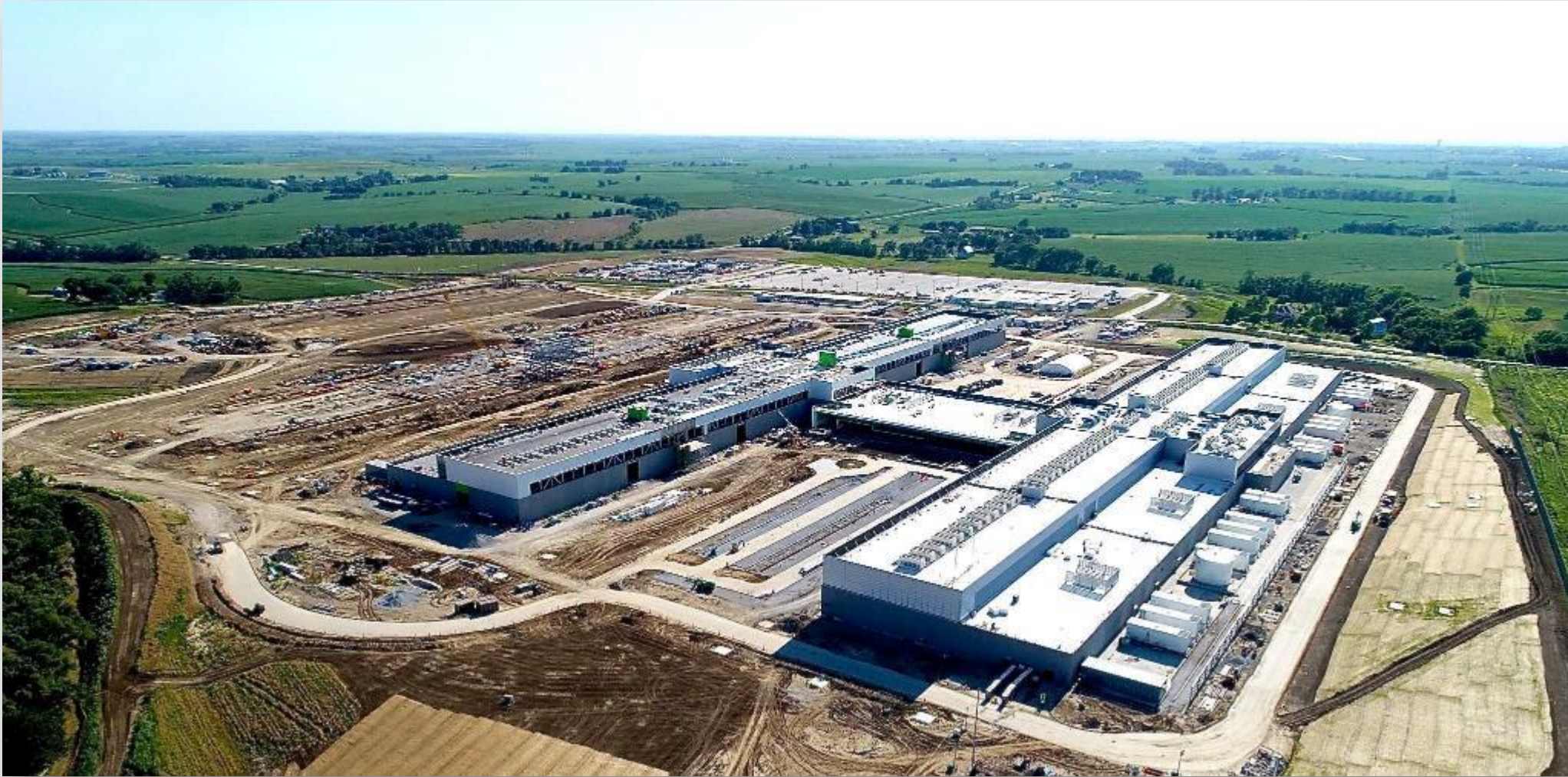
Facebook Data Center. 1,000-plus contractors currently on-site.
