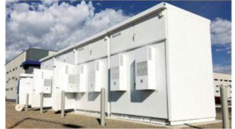
Example of 1 MW, 2hr (2 MWh) battery
