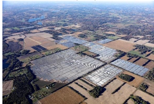
NorthStar Solar (MN)–100 MW
